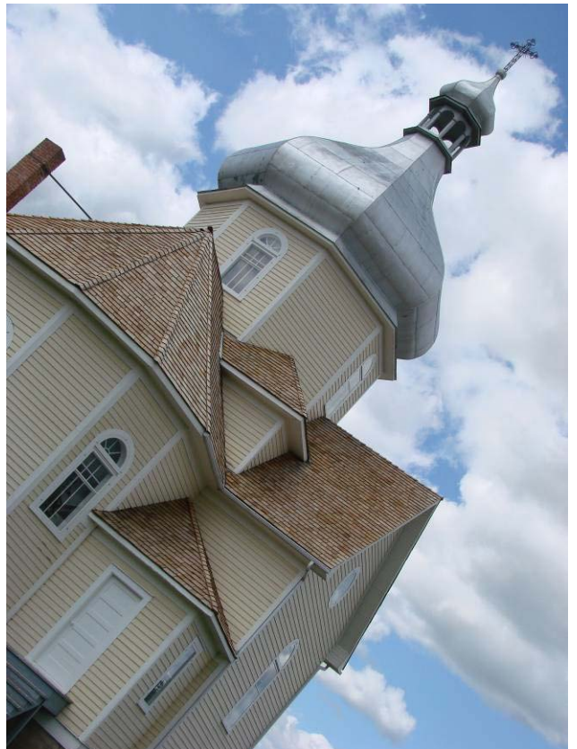
Close up of East Side
